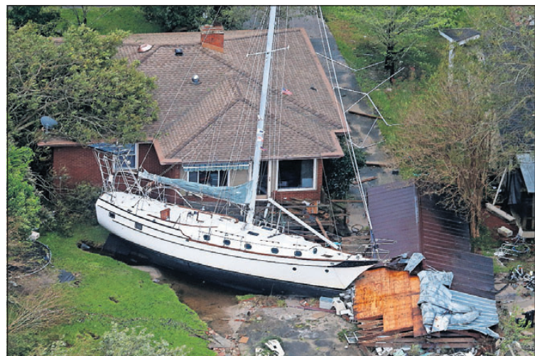
A sailboat is shoved up against a house and a collapsed garage Saturday after Florence, now a tropical storm, blew through New Bern, N.C. [STEVE HELBER/THE ASSOCIATED PRESS]
